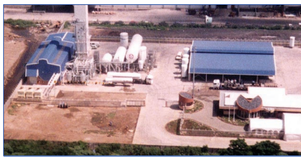
Figure 3. Costain designed cryogenic air separation unit.
